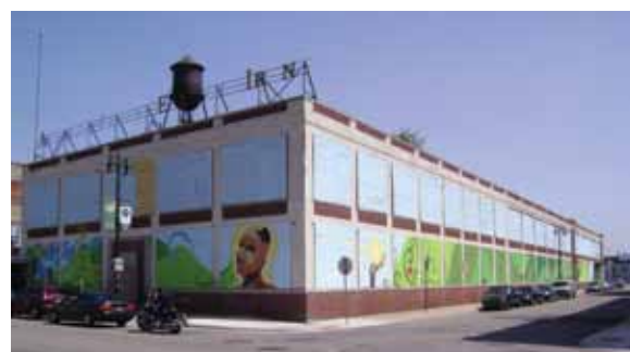
Interior contents, building materials and murals at the former American Beauty Electric Iron building in TechTown were reused, recycled and relocated by Wayne State.
